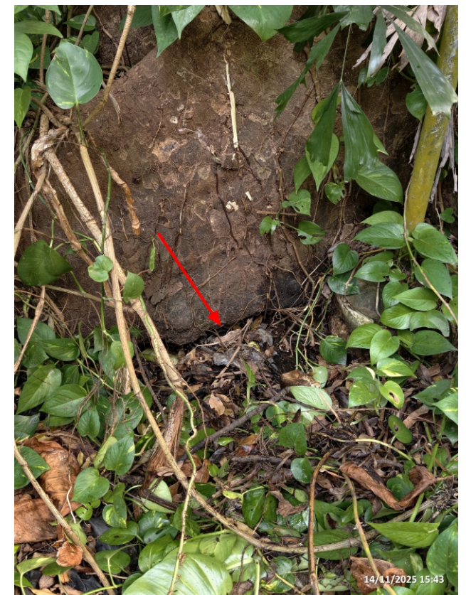
T08 (F) - Cavity under Trunk Base and Full of Water
